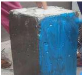
Saturant is applied with column surface
