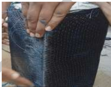
C.F is wrapped to the surface
