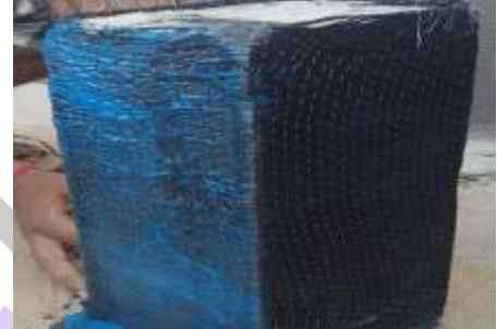
One more coat saturant is applied
