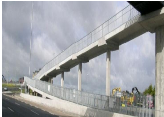
FIG 4.3- Reinforced Concrete Footbridge
