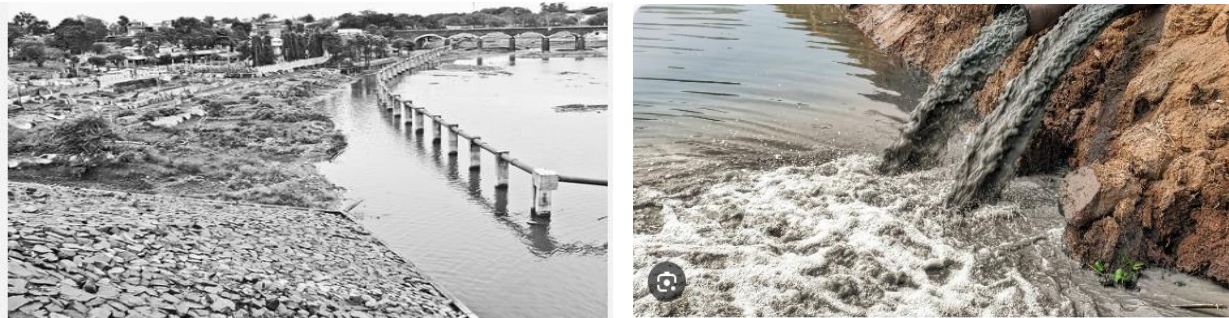
Figure 5 Waste Disposal River Side and Flowing Drain
