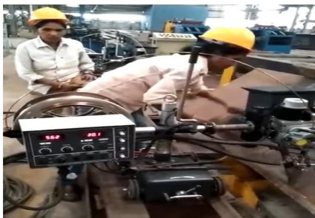
Figure 4: Submerged Arc Welding Machine in experiment
