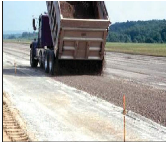
Fig.5 Spreading of excess aggregate for formation in FDR procedure.
