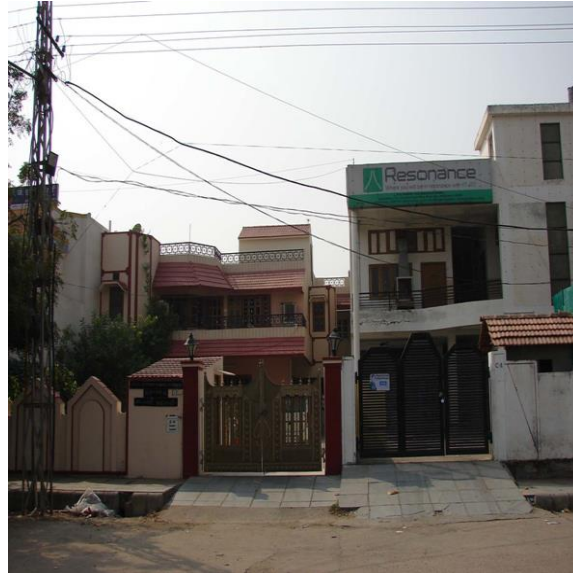
Fig 3: Residential houses, Dadabari
